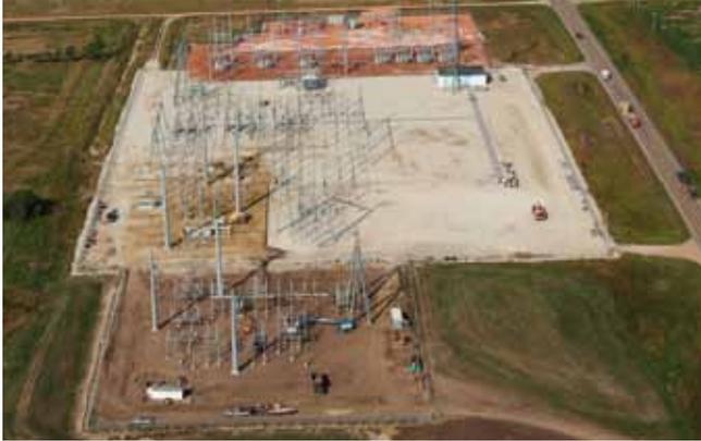
The Charlie Creek Substation near Killdeer is getting a new transformer and a 230-kilovolt bus. The additions support Western's upgrade of their line that heads north out of the substation.
