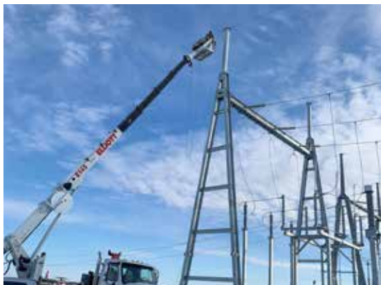
The final span of fiber being pulled at the Neset substation.
