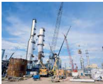
Workers assemble the original ammonia towers in 1996.
