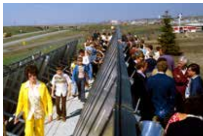
A tour of the 270 double glass solar collectors at Headquarters in 1978.
