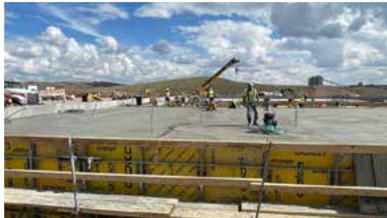
Concrete being poured near Dry Fork Station.
