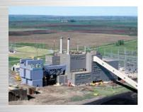
The first biomass system in a lignite coal-fired boiler was commissioned in 1982 at the William J. Neal Station near Velva, North Dakota. The boiler was modified to burn sunflower seed hulls.
