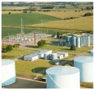
Spirit Mound Station was the first Basin Electric generating facility in South Dakota, commissioned in 1978. The two 60 MW oil-fired combustion turbines provide 120 MW of electricity, primarily on an as-needed basis. The facility can be remotely operated.
