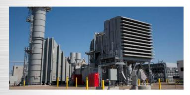
Groton Generation Station Unit 1 near Groton, South Dakota, was the first commercial application of General Electric's LMS100° simple-cycle turbine technology. It went into commercial operation in 2006. Unit 2 also employs the same technology.
