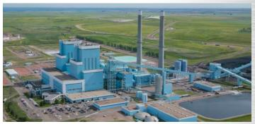
Antelope Valley Station's boilers were the largest in physical dimensions of any others in the world at the time of construction.
