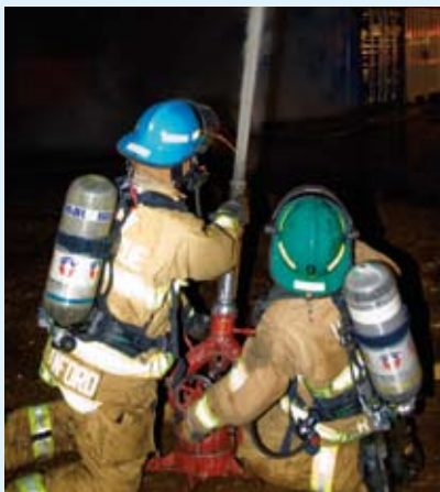
Fire fighters from Stanton and Hazen responded to quickly suppress the fire at the scrubber construction site.
