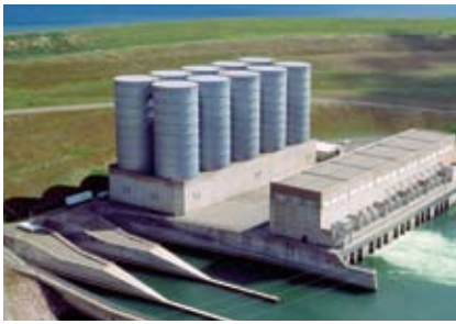
Western's power comes from dams like the Garrison Dam in North Dakota.
