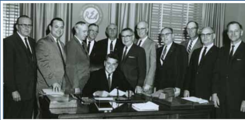
May 10, 1962: REA Administrator Norman Clapp (seated) signs papers for a $36.6-million loan to construct the Leland Olds Station Unit 1, Basin Electric’s first power plant.
