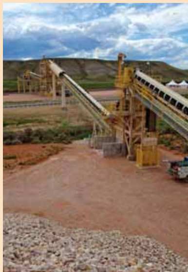
Limestone unloaded at the truck dump is conveyed across the highway to bins where it's loaded into rail cars.
