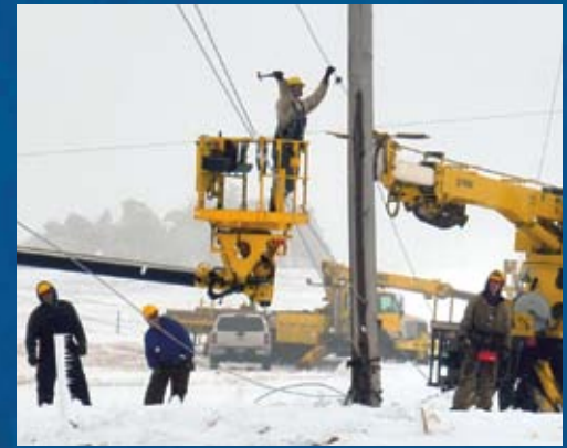
Corn Belt Power crews knock ice off power lines southeast of Sac City on Jan. 22. (Photo by Marena Fritzier of Corn Belt Power.)
