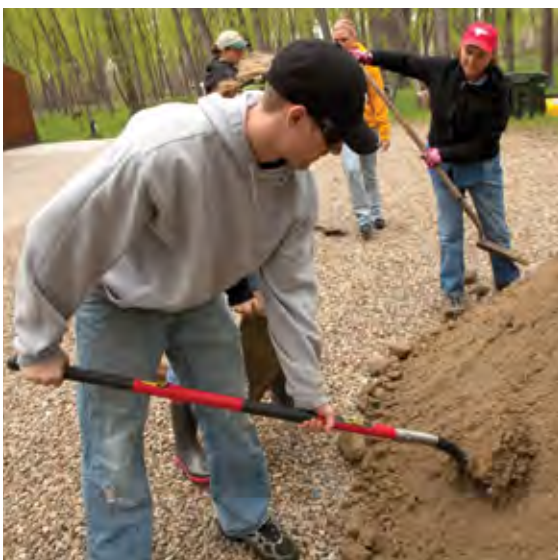
Mike Perreault, utilities field technician at Dakota Gasification Company, helps fill sandbags to protect the home of Mike Eggl, senior vice president of External Relations & Communications.
