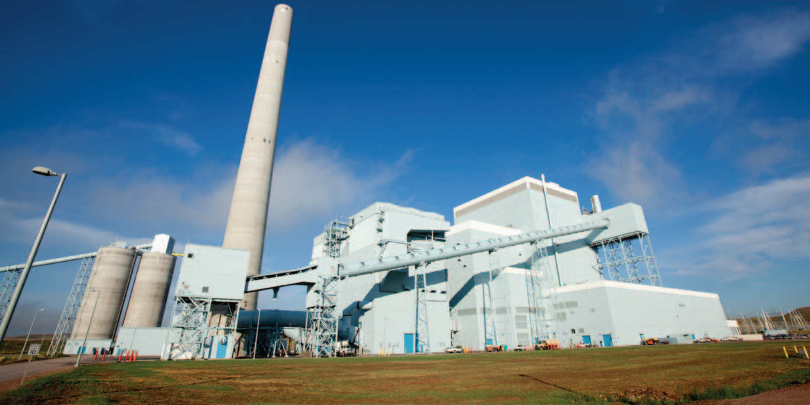
The power plant was built near the Dry Fork Mine to implement the mine-mouth model of operation. The coal is delivered from the mine to the power plant via a conveyor less than one mile in length.
