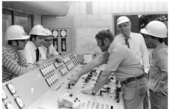
(From left) Basin Electric's Robert Boettcher, Kent Janssen, Richard Fockler, Vern Smith, James Grahl and Brown-Boveri Corporation's Didier De Vulpilleres watch the initial turbine roll at Leland Olds Unit 2 in 1975.
