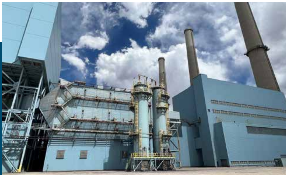
Laramie River Station uses environmental controls such as wet and dry scrubbers to reduce emissions. The technology helps ensure the air we breathe remains safe and clean.
